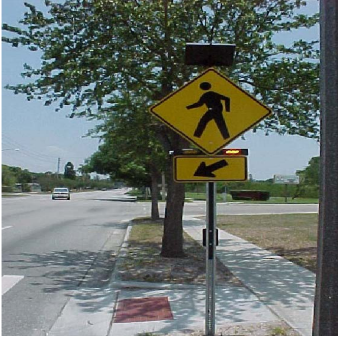
Figure 1. Photo. RRFB with two forward-facing LED flashers and a side-mounted LED flasher.
