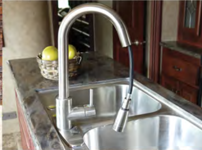
Residential stainless double-bowl sink with high-arch pull-out sprayer faucet.
