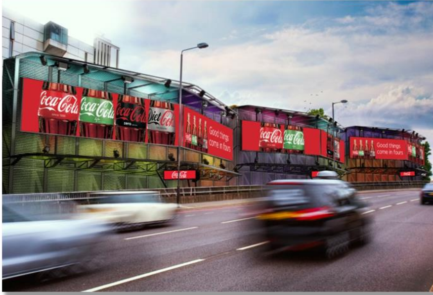
(Figure 3 – Ultravision’s UltraPanel forming the largest digital display in Europe)
