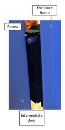
35. The hinges that were removed from the RMR Enclosure further infringe claims 8 and 15 of the '396 Patent because, as shown in the annotated photographs above and below, the mounting holes of the hinge do not extend completely through to the front of the hinge portions.
