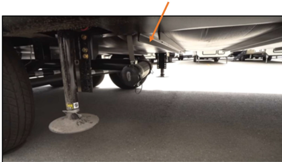
Exemplary beam located in the 3 rd section (beneath the garage)
