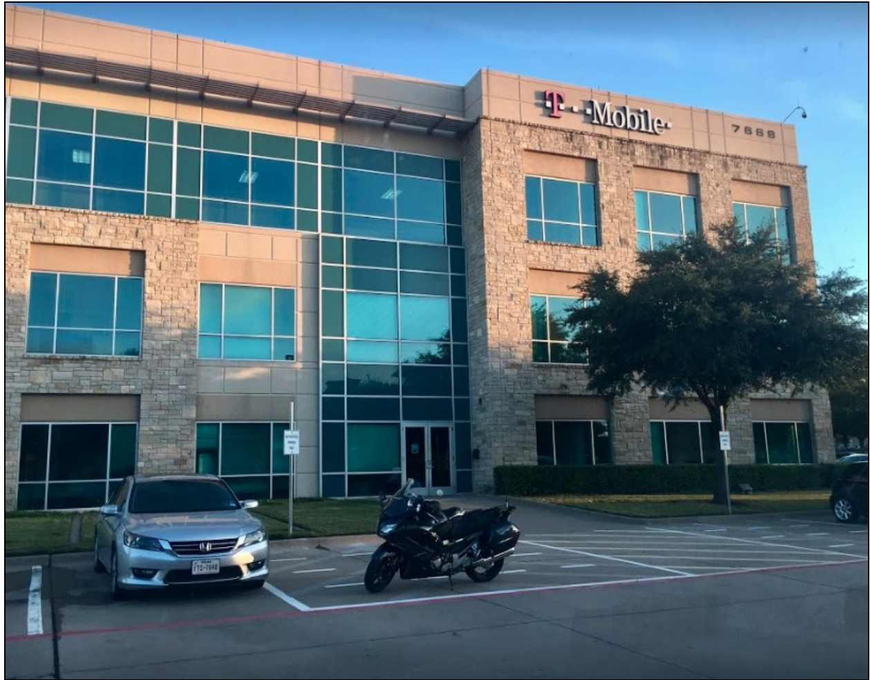
Fig. 1: Depicting T-Mobile office at 7668 Warren Parkway, Frisco, TX.
