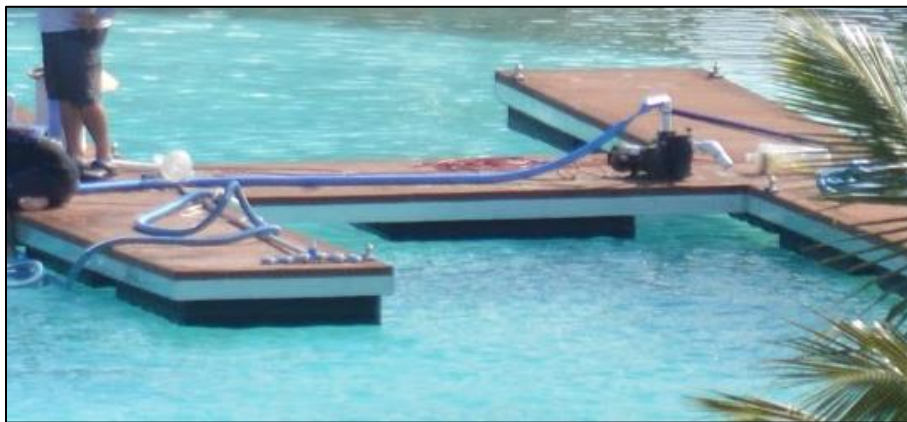
Figure 25: Pumping system connected to a moveable suction device cleaning the sloped walls
