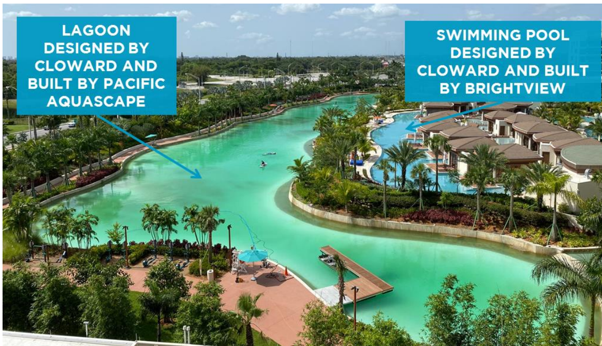
Figure 8: Hard Rock Swimming Pools and Lagoon, pools constructed by Brightview and the Lagoon constructed by Pacific Aquascape
