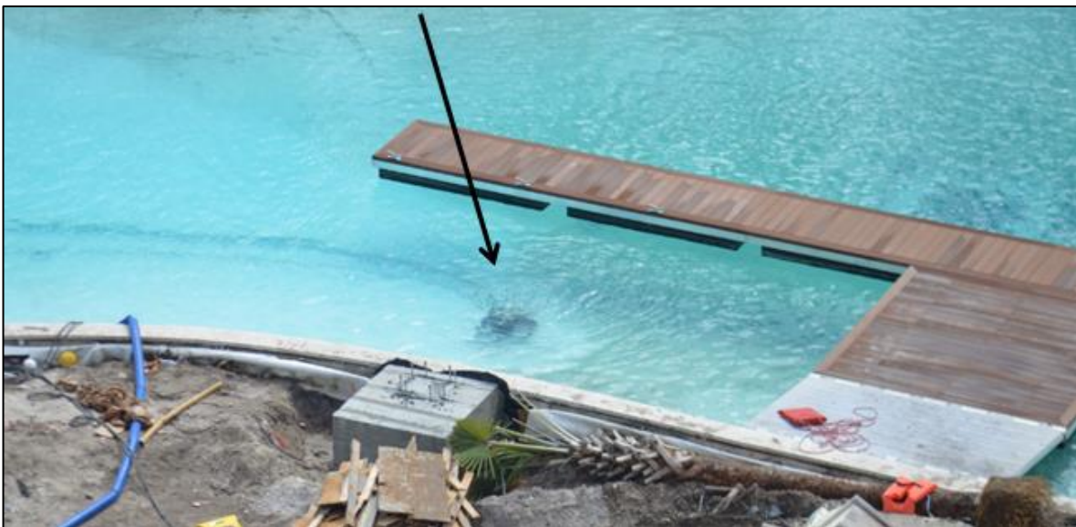
Figure 20: Diver performing manual cleaning using a moveable suction device in the sloped walls
