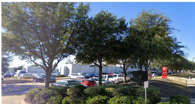
Tesla Gallery and Service Center located at 5800 Democracy Drive, Plano, Texas, 75024
