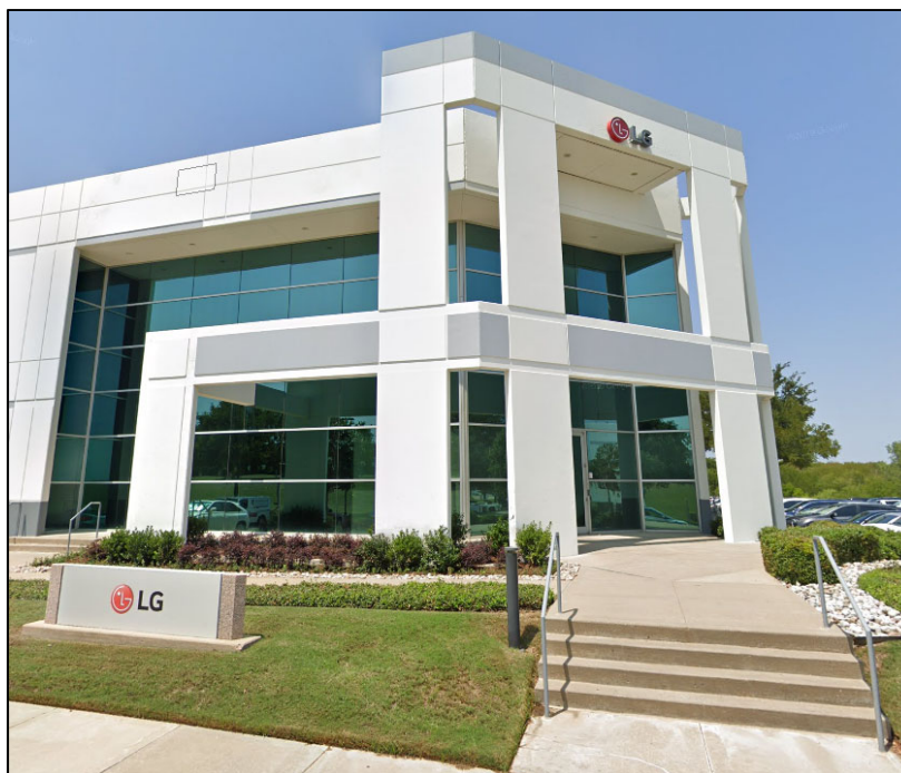
LG's Facilities at 2153 and 2155 Eagle Parkway, Fort Worth, Texas.
